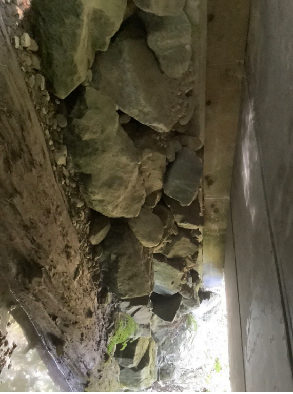
Left Bank Abutment when facing downstream
