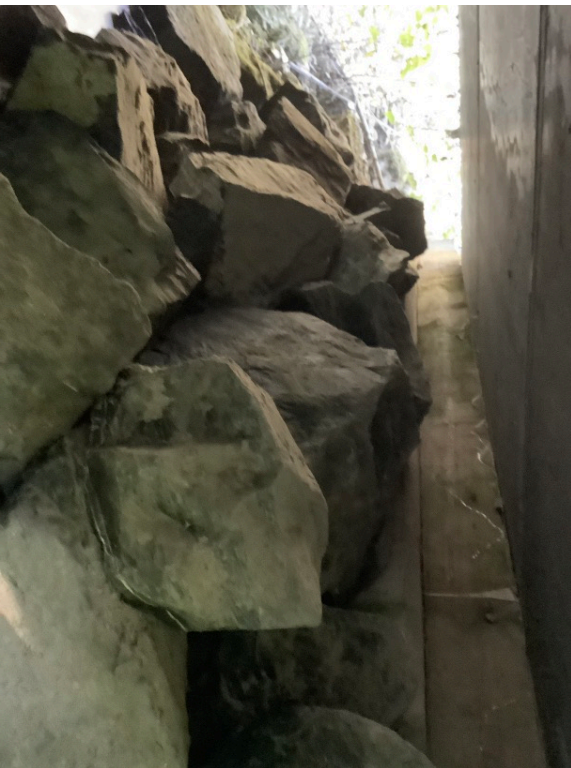
Right Bank Abutment when facing downstream
